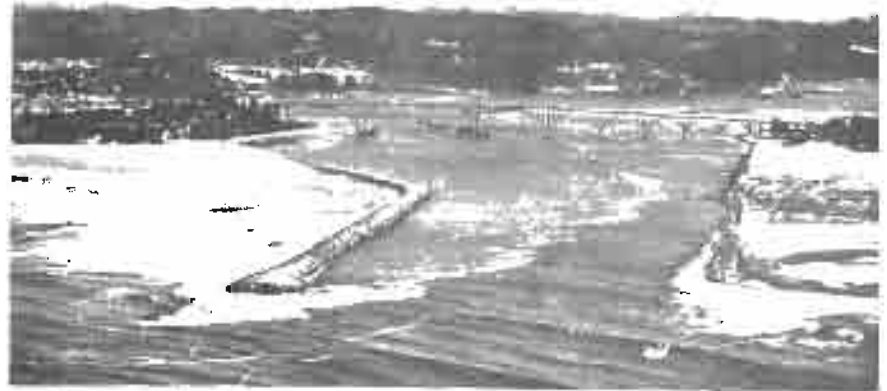
North jetty at Yaquina Bay is being extended 1,800 feet in a $5,376,000 project.
