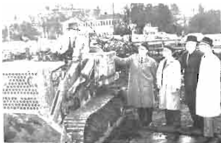
DR. WAYNE V. BURT DRIVES CAT FOR GROUND-BREAKING CEREMONIES FOR THE NEW OCEANOGRAPHY BUILDING ON OREGON STATE UNIVERSITY CAMPUS. SECOND FROM RIGHT IS DR. JAMES JENSEN, PRESIDENT OF OSU.
